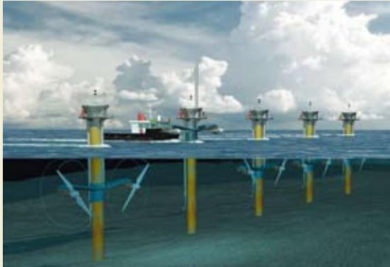
7.12 b > Tidal energy can be converted to electricity by underwater rotors, as at the SeaGen plant off the coast of Northern Ireland in Strangford Lough. One facility has already been constructed which feeds electricity into the grid onshore. Others will follow.
